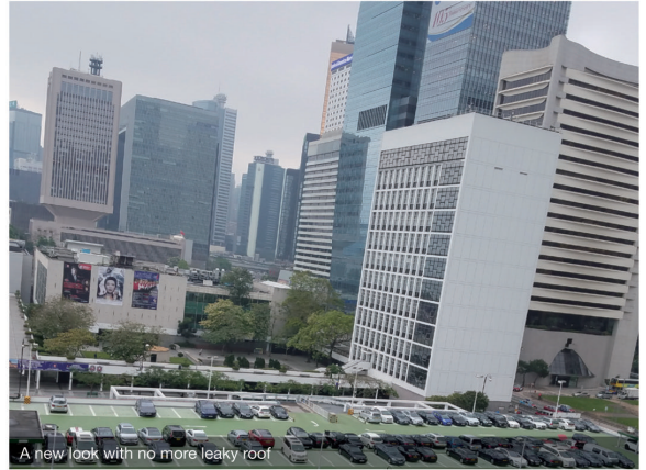
A new look with no more leaky roof
