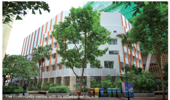
The community centre with its refurbished façade
