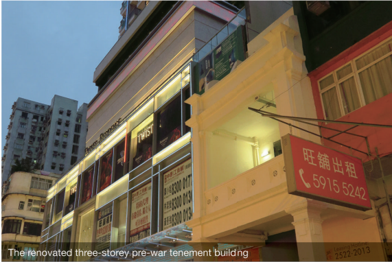
The renovated three-storey pre-war tenement building
