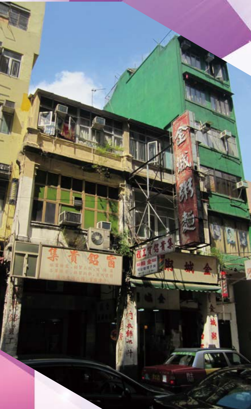
3-storey pre-war tenement building at 103-105 Parkes Street, Kowloon
