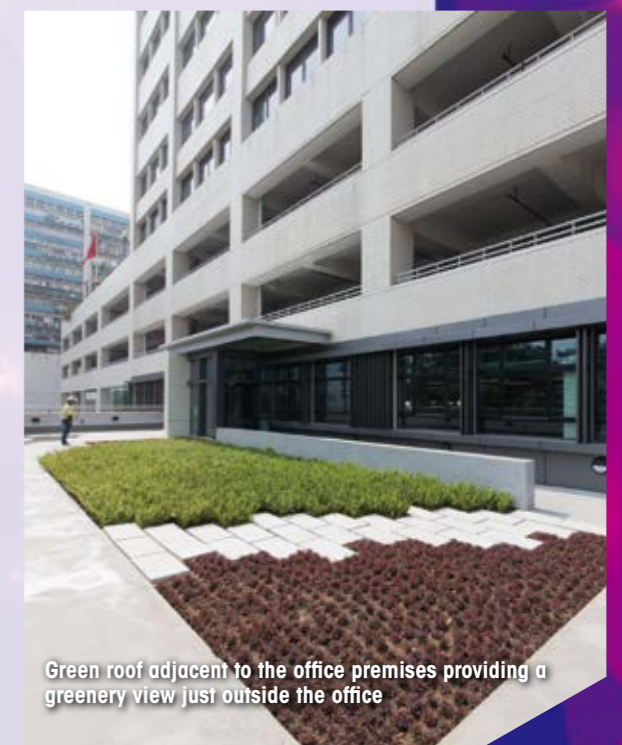
Adoption of innovative designs such as radiant cooling system, indirect LED lighting and sustainable materials
